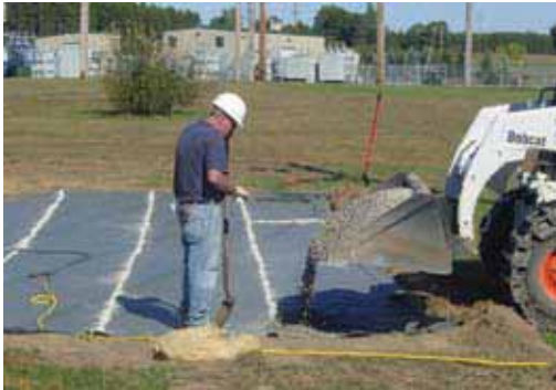
Bentonite is placed over the seams. Gravel is then placed over the material.
