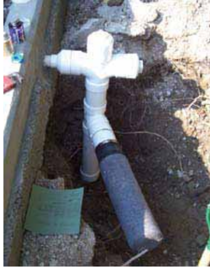
Wall mount install.
