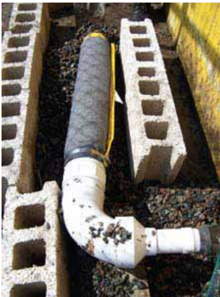
Pad mount install.
