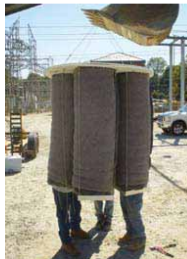
Catch basin drain filters.
